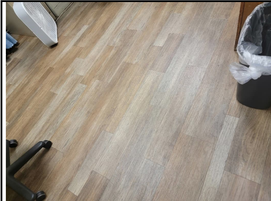
29. Assumed ACM Vinyl Sheet Flooring in Security Office
