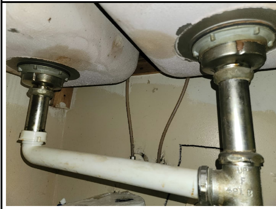
28. Assumed ACM White Undersink Coating
