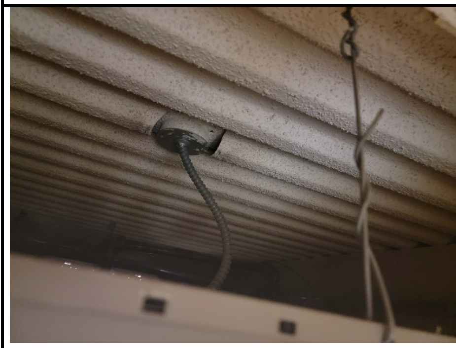
24. ACM HA 6 – Ceiling Texture on Metal Decking above Ceiling Tiles
