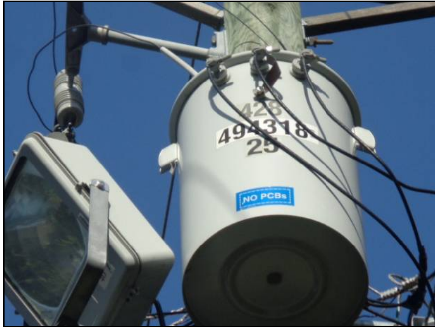
21: View of the on-site pole-mounted electrical transformer
