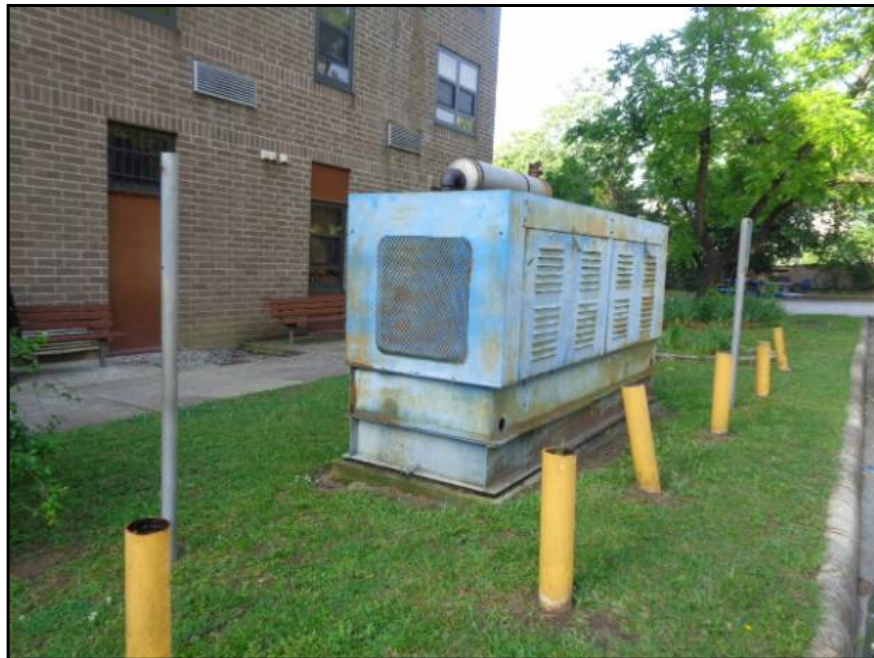
18: View of the out of use emergency generator and associated approximately 700-gallon diesel aboveground storage tank (AST)
