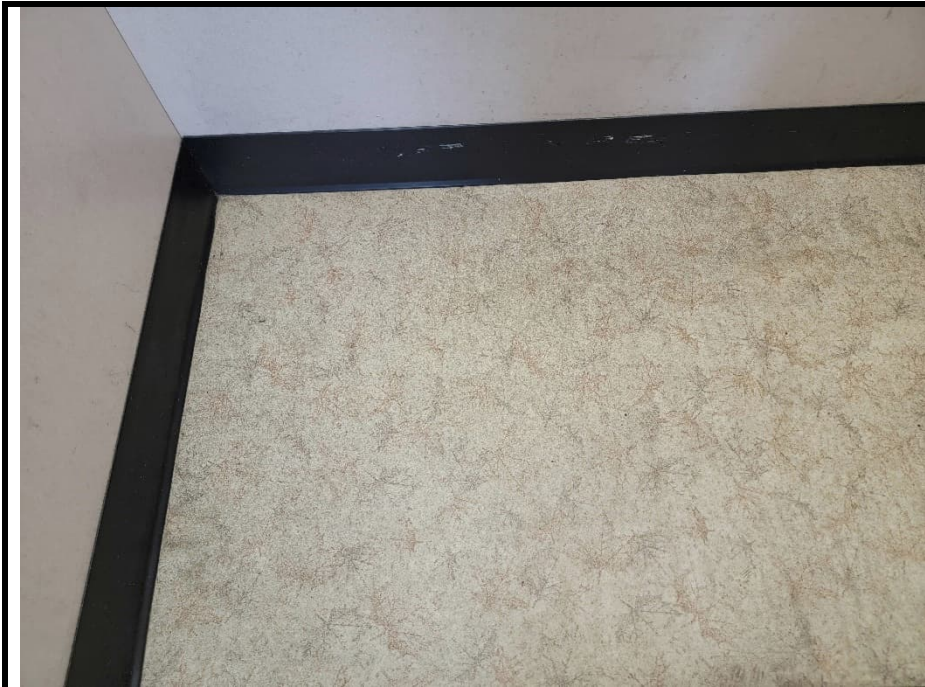
31. Assumed Vinyl Sheet Flooring and Assumed 6" Cove Baseboard in Elevator
