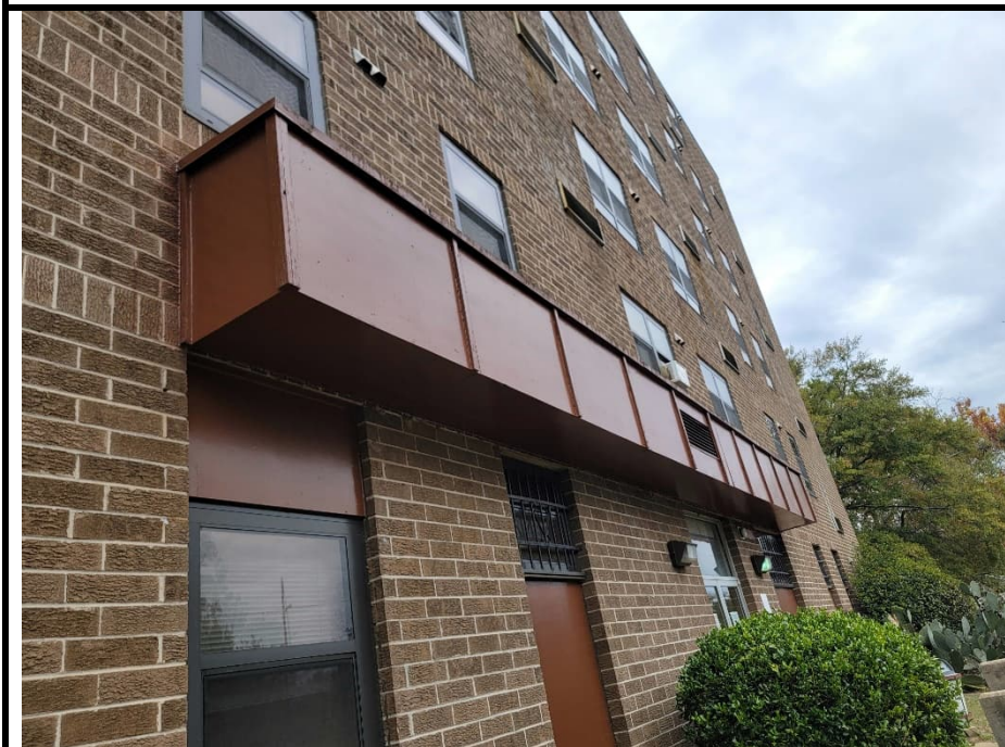
36. Assumed ACM Transite Panels on Exterior
