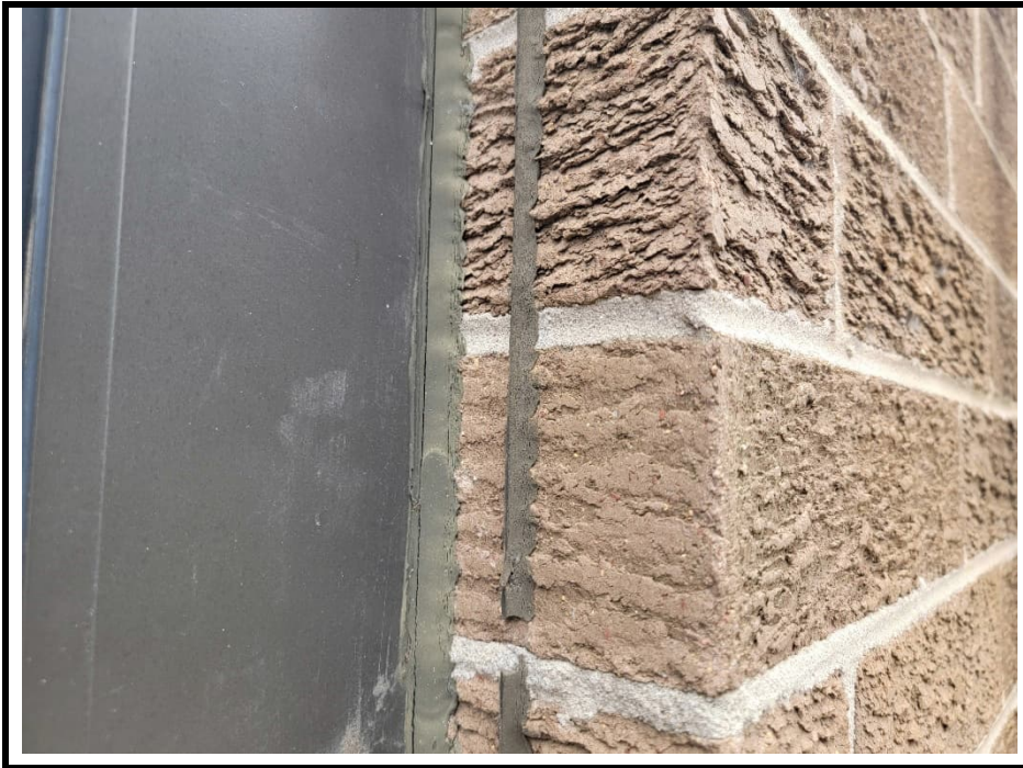
37. Assumed ACM Exterior Window Caulking
