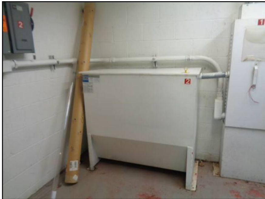
16: View of the on-site hydraulic elevator equipment
