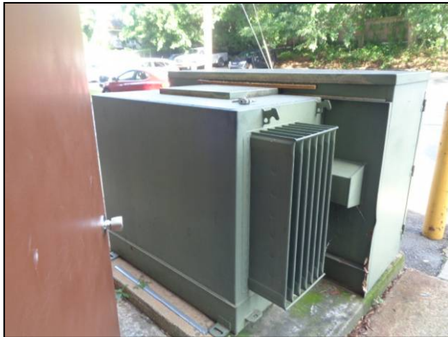
22: View of the on-site pad-mounted electrical transformer
